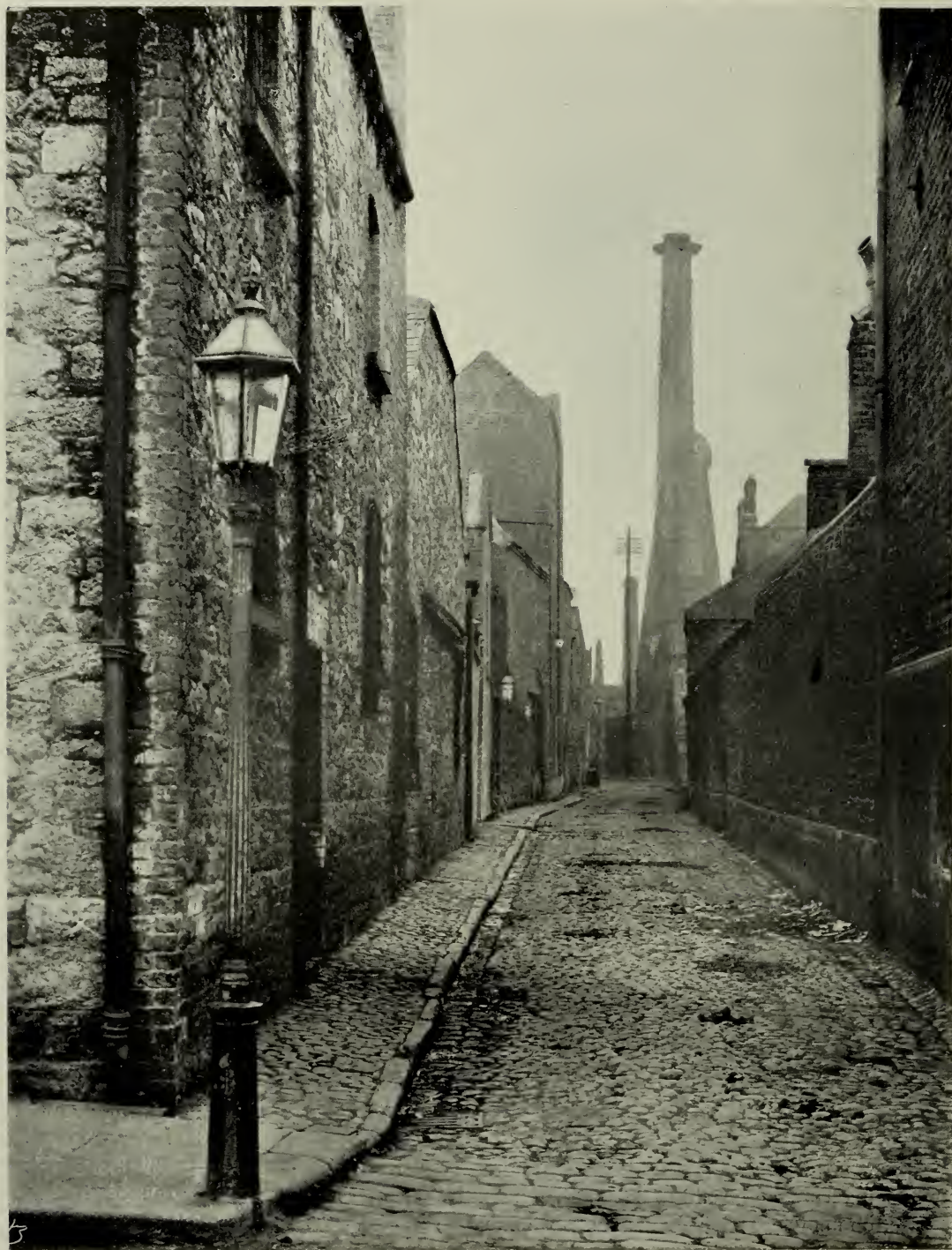
MARSHALSEA-LANE, THOMAS-STREET. Site of Robert Emmet's principal depôt in 1803.
